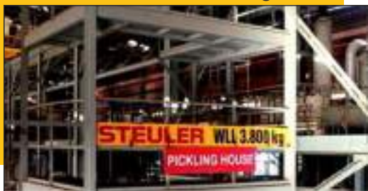
STEULER Pickling Plant
